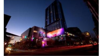
Block 21 (pictured) is the first mixed-use high rise tower in Austin to receive the USGBC LEED (Leadership in Energy & Environmental Design) silver certification
